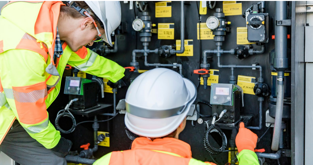
A meter billing service provider switches from yearly manual reading to the use of wM-BUS based heat cost allocators and a smart meter gateway.
